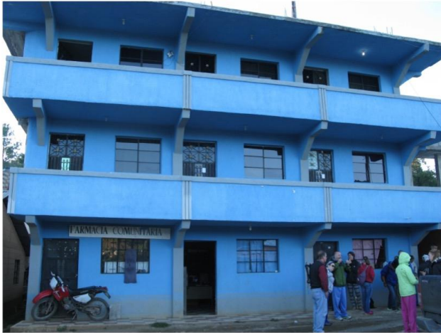
The Volunteer Building - built by Impact Global Health Alliance Volunteers!
